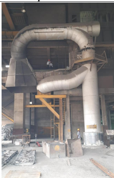
Stack attached to RABH-Reverse Air Bag House (2No's) in Ferro Alloy Division.
