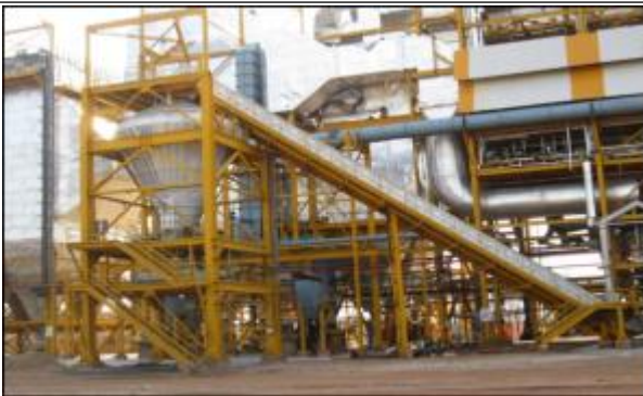
Stack attached to RABH-Reverse Air Bag House (2No's) in Ferro Alloy Division.
