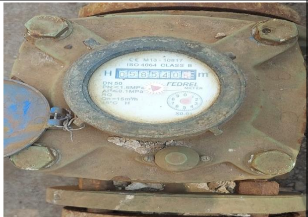
Power Plant Blow down water flow meter
