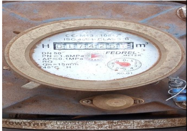
Power Plant Blow down water flow meter
