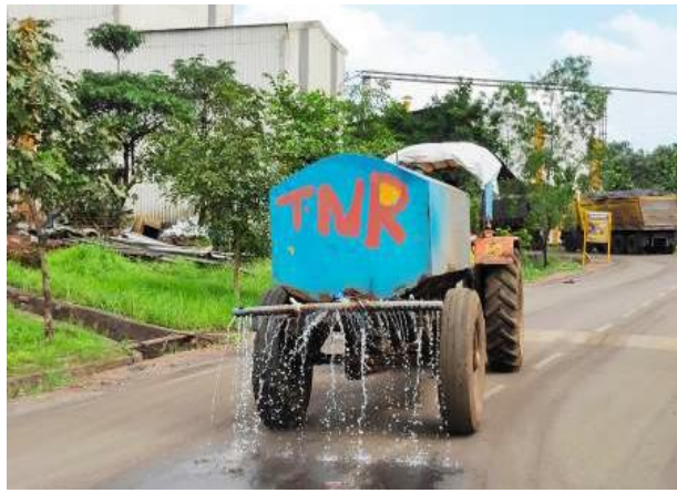
Water Sprinkling System & Haulage Road Dust Suppression
