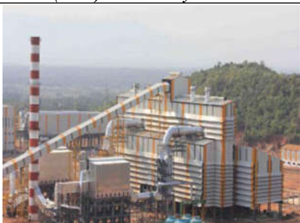
Stack attached to RABH-Reverse Air Bag House (2No's) in Ferro Alloy Division.
